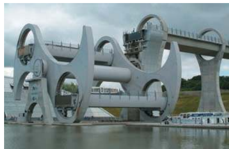
FIGURE 13.19 The Falkirk Wheel has two balanced water-filled gondolas, one going up and one going down. The gondolas rotate as the wheel turns, so the water and boats don't tip out.
