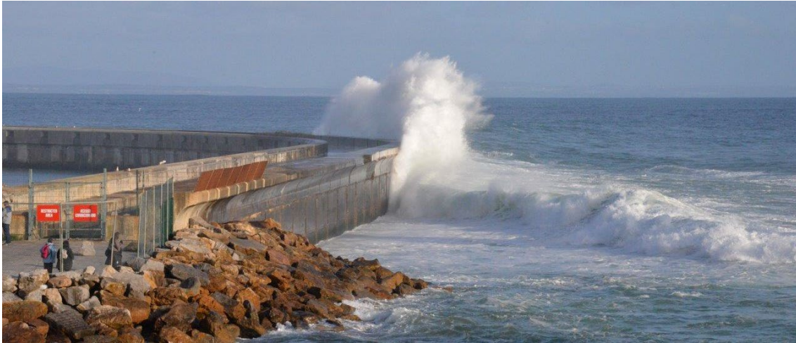
Figure 1.11: Effective fairly significant bullnose at Cascais, Portugal. Waves are breaking on the foreshore and give impulsive wave conditions. There was no wind. Courtesy L. Franco
