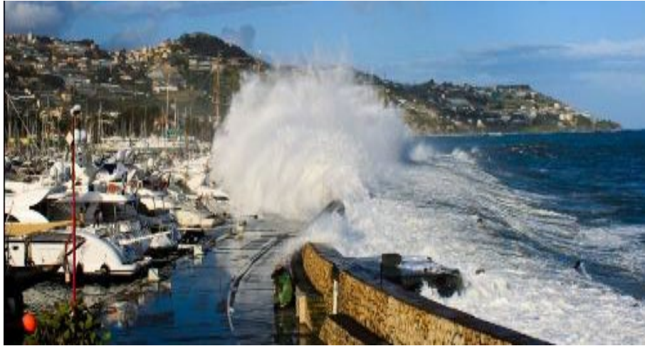
Figure 3.12: Wave overtopping at the marina of San Remo, Italy, damaging small boats
