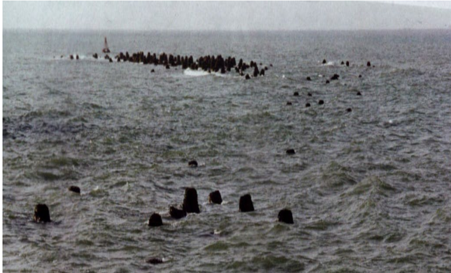
Figure 3.11: Remains (tetrapods) of a breakwater failed by wave overtopping, destroying the rear side of the structure and then a full collapse of the crest. Porbandar, India
