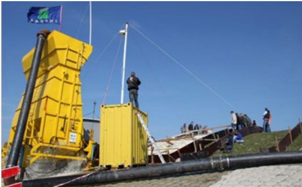
Figure 4.38 Pilot wave run-up test at Tholen, using the existing Wave Overtopping Simulator
