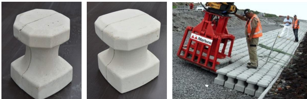
Figure 5.27: Impression of Hillblocks®. Left: type 'Slim', middle: type 'Basic', right: during placing procedure on a dike. Courtesy Deltares
