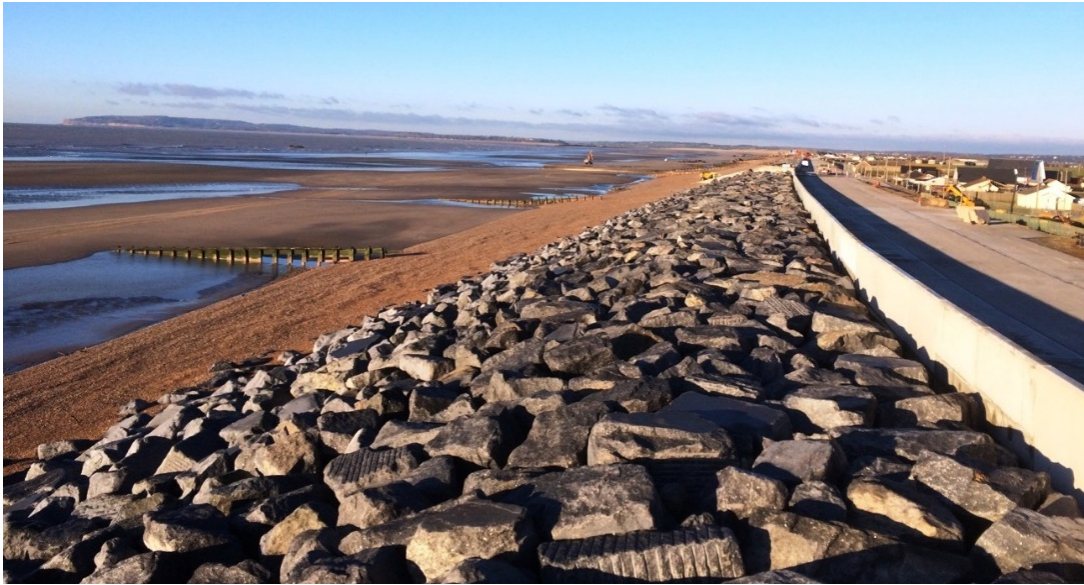
Figure 8.8: Broomhill Sands revetment
