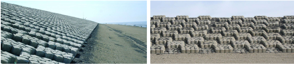
Figure 5.31: Chessboard pattern produced with two thicknesses of placed block revetments. The roughness has only been placed in the run-up zone, above the wide asphalt berm
