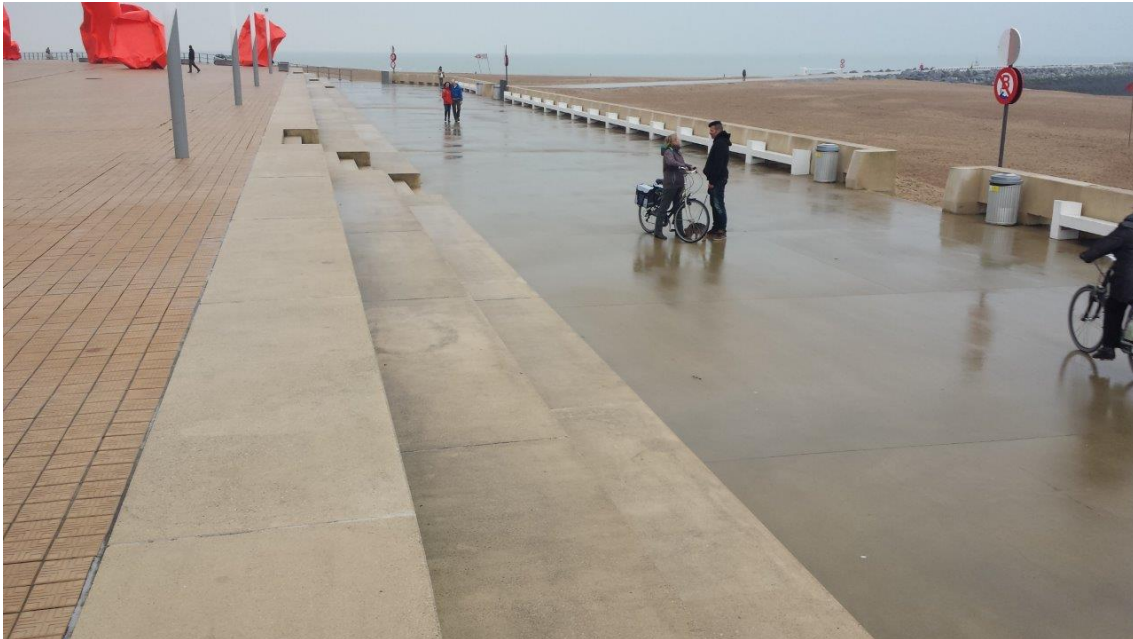
Figure 5.52: A stilling wave basin at Oostende, BE
