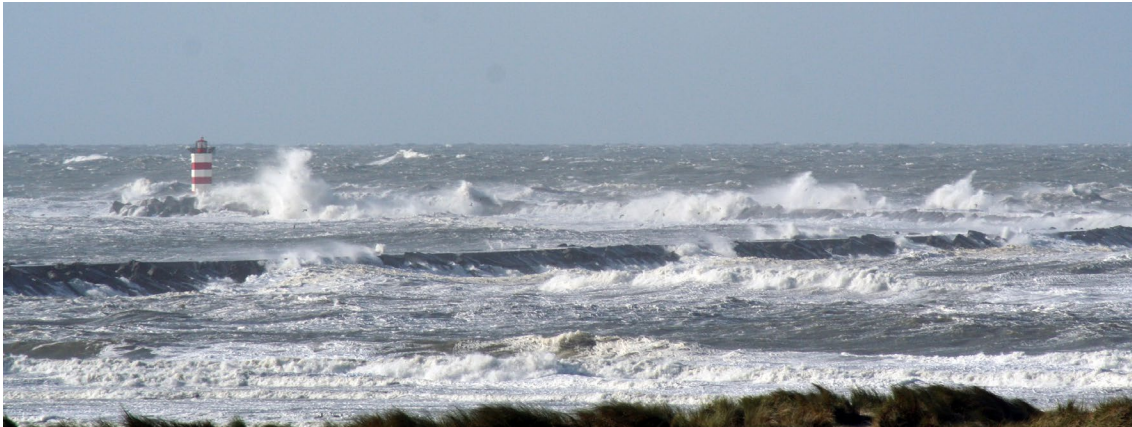
Figure 4.12: Wave overtopping and transmission at breakwater IJmuiden, the Netherlands
