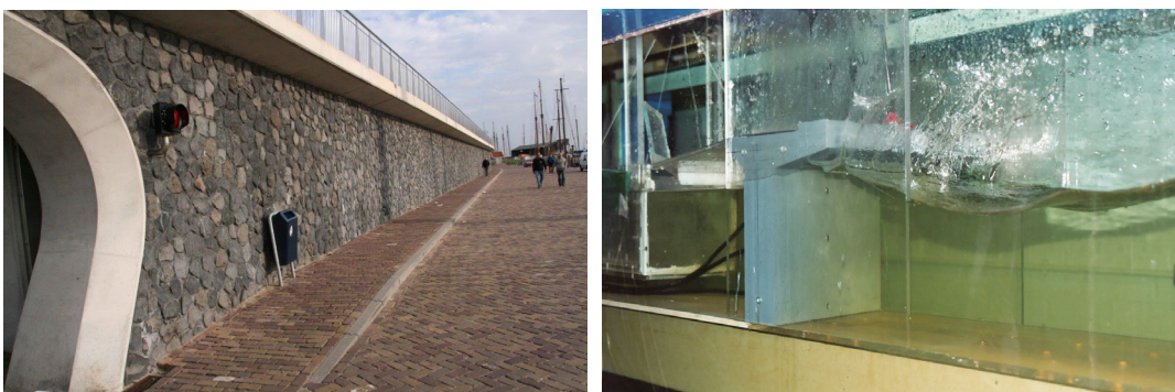
Figure 1.12: Large and effective wave return wall at Harlingen (NL). The wave return wall is part of a promenade on top of the wall (picture above). Lower left: the wall with wave return wall in reality; lower right: model testing under design wave conditions
