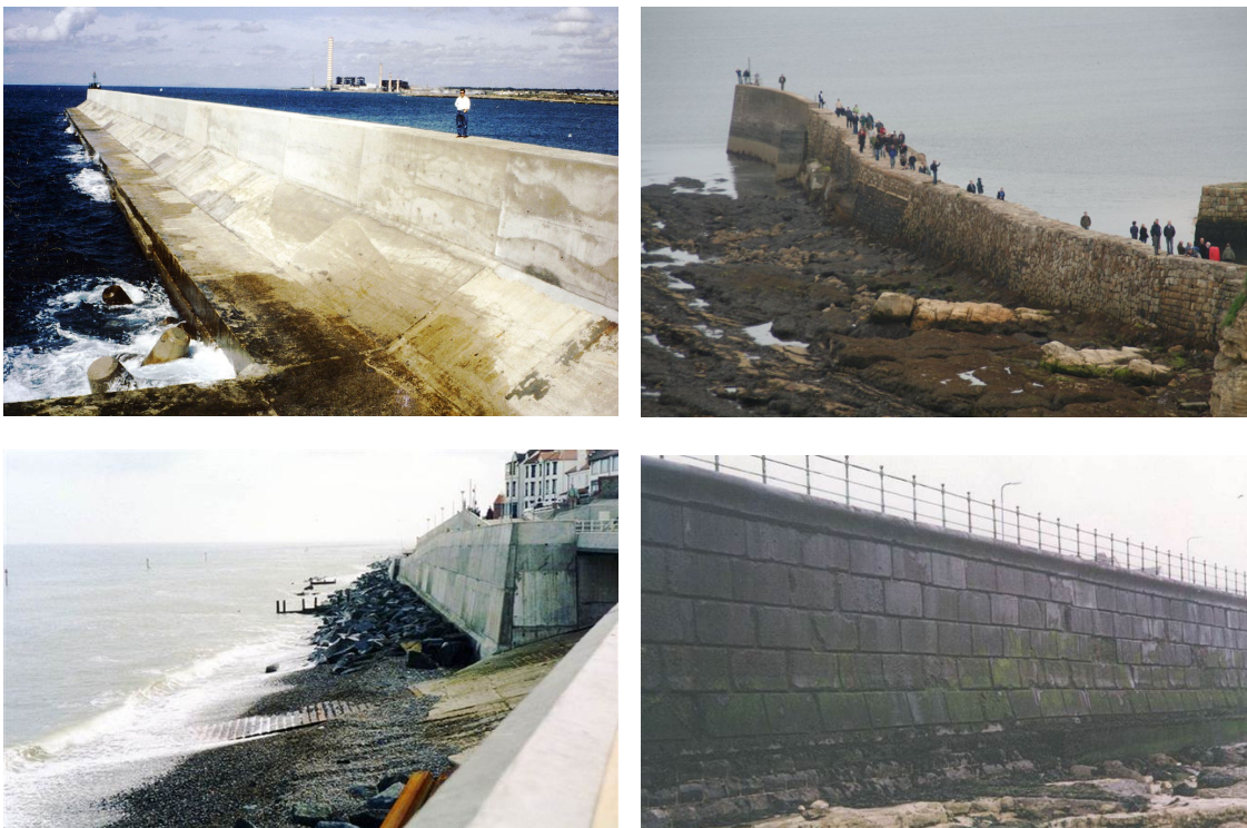
Figure 7.1: Vertical structures: (clockwise top left) modern caisson breakwater with shifted parapet (Civitavecchia, Italy), old blockwork breakwater (St Andrews, UK), modern concrete seawall and older stone blockwork seawall with bull nose
