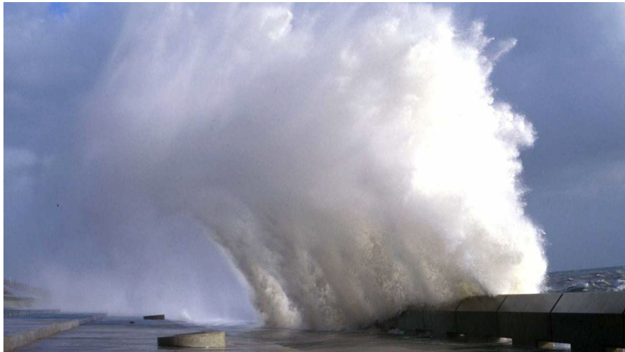
Figure 3.17 Severe wave overtopping at Samphire Hoe, UK.
