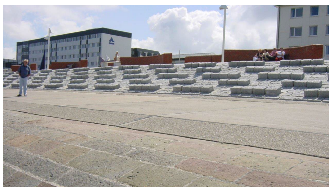
Figure 5.26: Example of battens or ribs in reality
