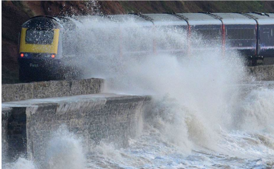
Figure 3.23: Wave overtopping onto a moving train, UK
