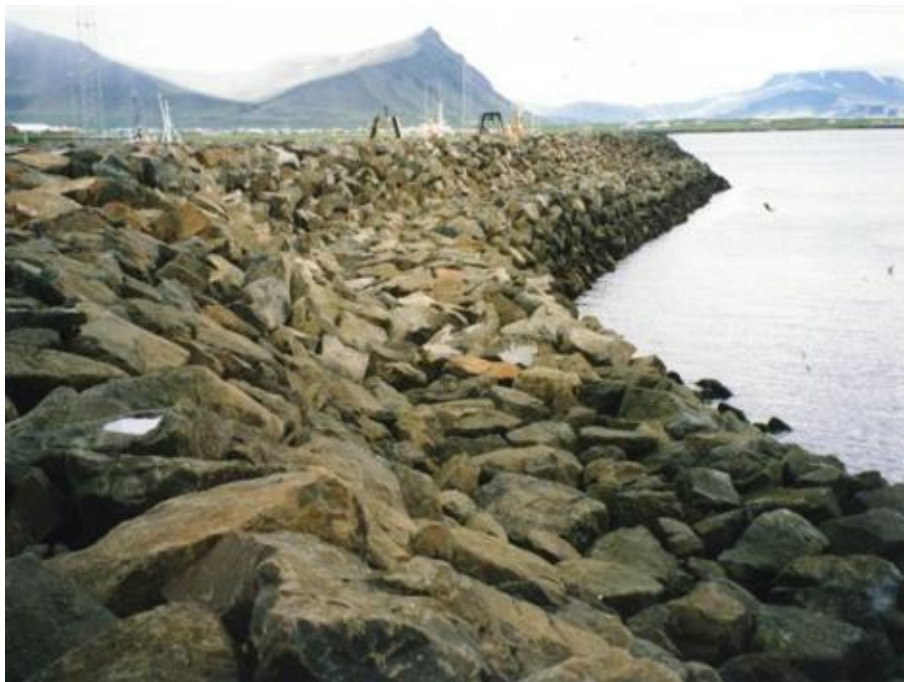
Figure 6.10 Icelandic-type berm breakwater
