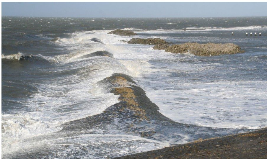
Figure 3.20 Dangerous overtopping over a smooth low-crested structure. Near locks at Afsluitdijk, NL
